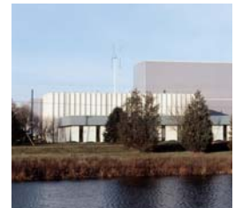
US center of excellence for food and dairy process equipment
