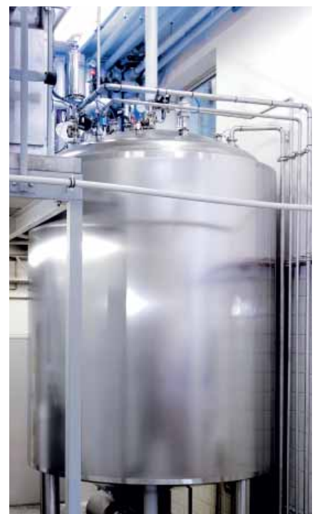
The Niro Pharma Test Station includes a validated purified water production and distribution system. The PW production unit supplies the spray dryer CIP and feed systems with water meeting the pharmacopoeial quality standard.
